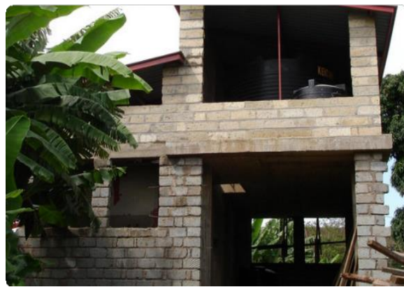
Clean water for the hospital in Nkubu, Kenya [2006-2007].
