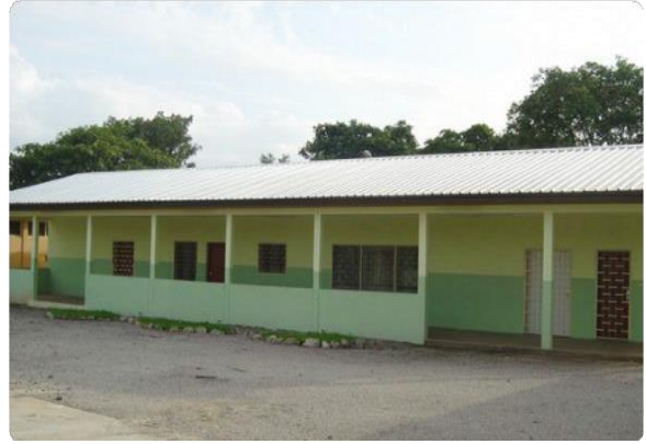
Hospital project, Bossemptélé, Central African Republic [2011-2013].
